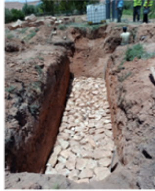
Foundation stabilization
